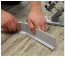
The inside and outside corners may be created from the profile using the Döllken punch. Installation will be invisible with the Döllken hot melt adhesive.
